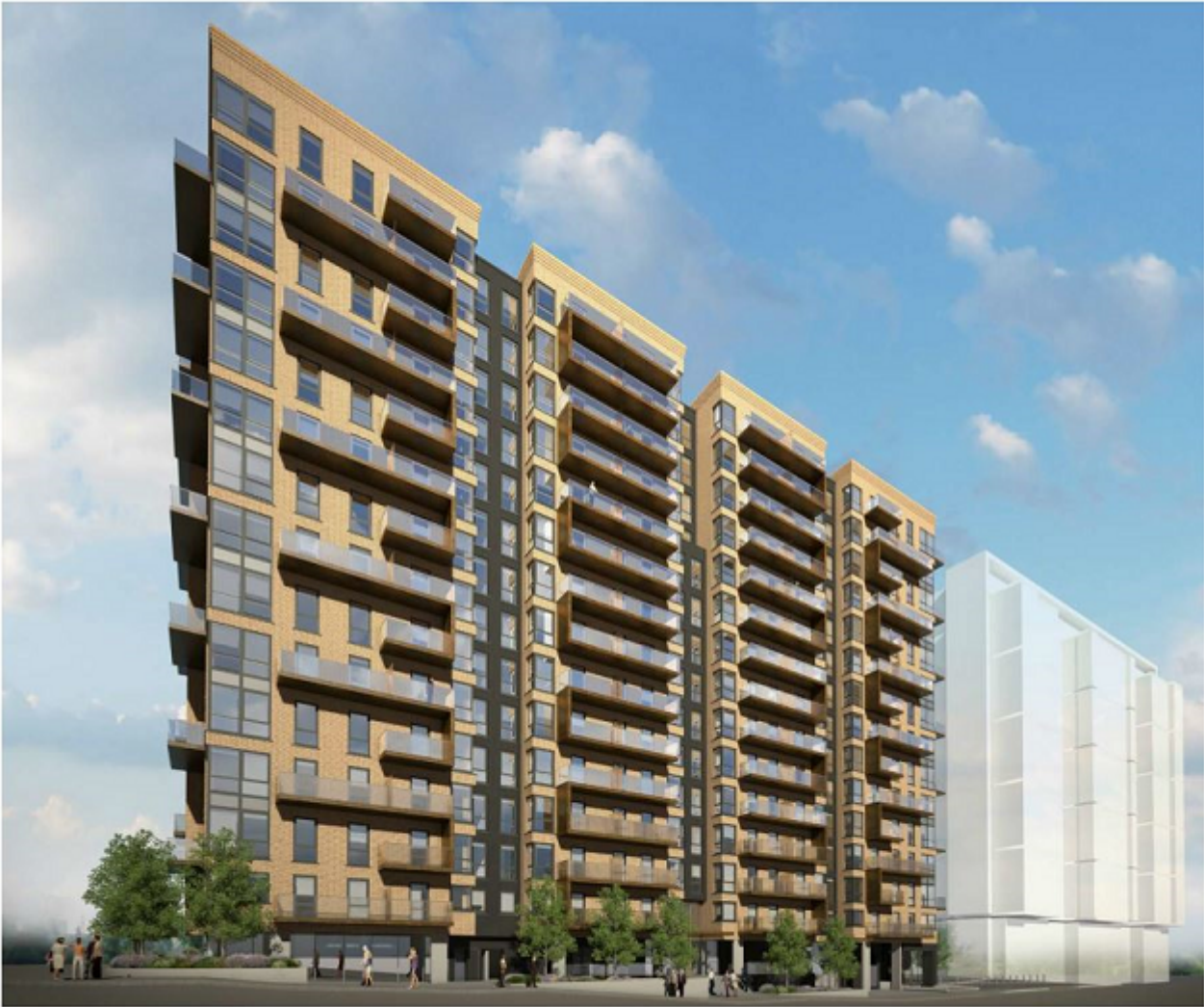
View looking down Rutherford Way
